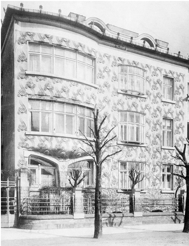
Figure 1. Langer House, Vienna
