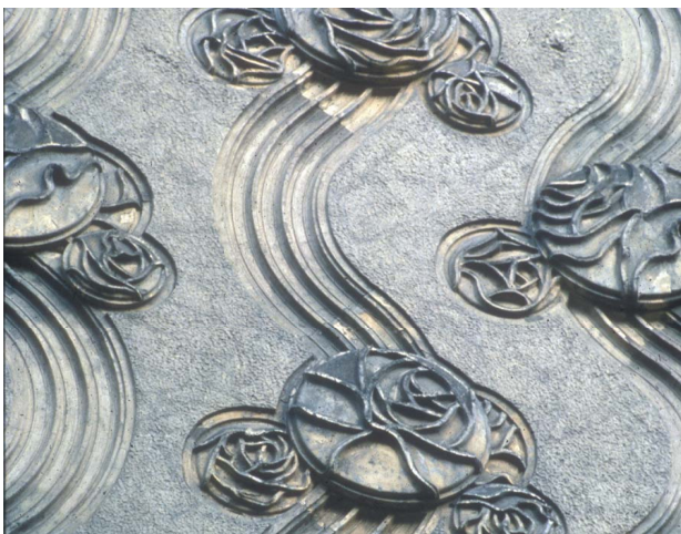
Figure 2. Langer House, Detail
