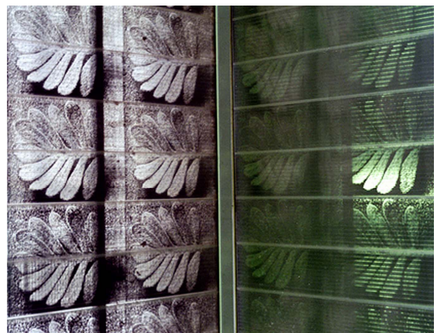
Figure 5. Ricola Storage Facility, view of printed wall and ceiling panels (photo A.Godel)
